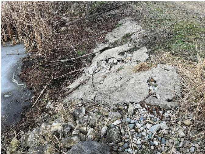
Photo 7: Inlet end of hydraulic outlet looking N. Buildup of vegetative debris around trash guard/riser structure and deteriorating concrete along slope between structure and perimeter road.
