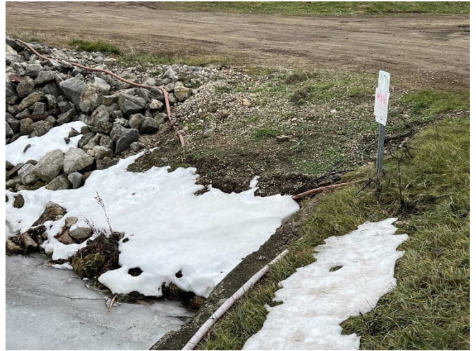
Photo 2: Soil covering riprap on outboard slope in NW corner.
