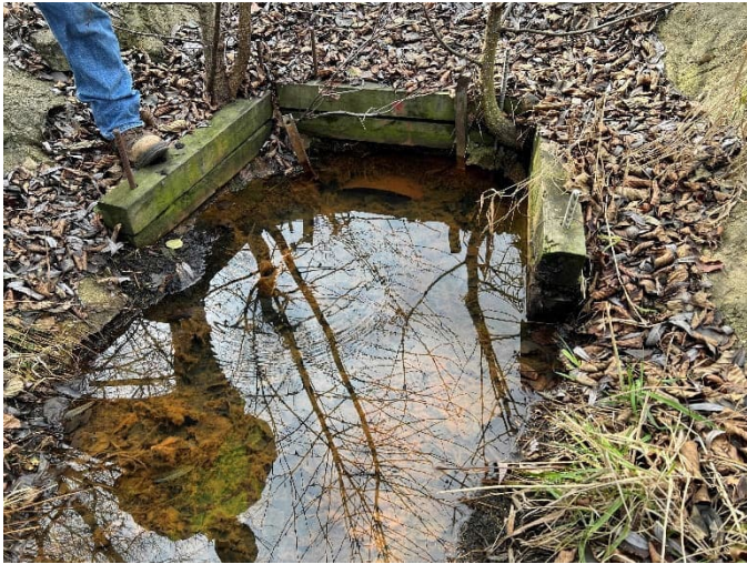
Photo 9: Outlet end of hydraulic outlet. No observable flow. Crown of pipe visible, submerged under lake water level. Debris buildup visible under water in channel from pipe to lake.
