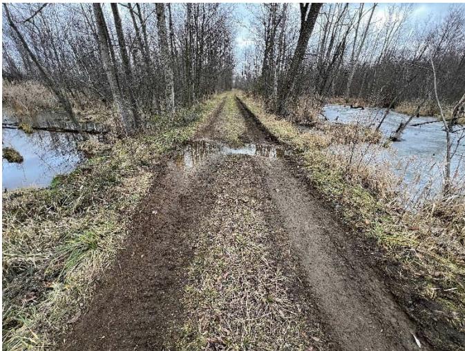
Photo 11: Road along southern perimeter looking E. Water flowing across road from south (right) to north (left). Vehicular rutting visible.
