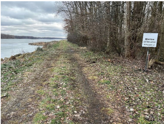
Photo 3: Road along northern perimeter looking E. Tall grass on outboard slopes (left side).
