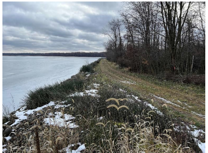
Photo 4: Road along northeast perimeter looking SE. Tall grass on outboard slopes (left side).
