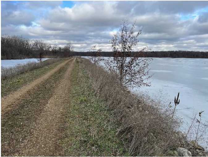
Photo 5: Road along eastern perimeter looking NNW. Several typical small trees and tall grass on slopes visible.
