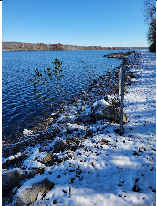
Photo 2: Road and outboard slope along north perimeter looking east. Vegetation on outboard slope.
