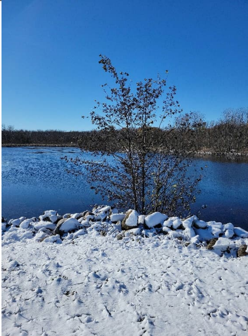
Photo 5: Road along eastern perimeter looking SW. Tall shrub/tree on inboard slope.
