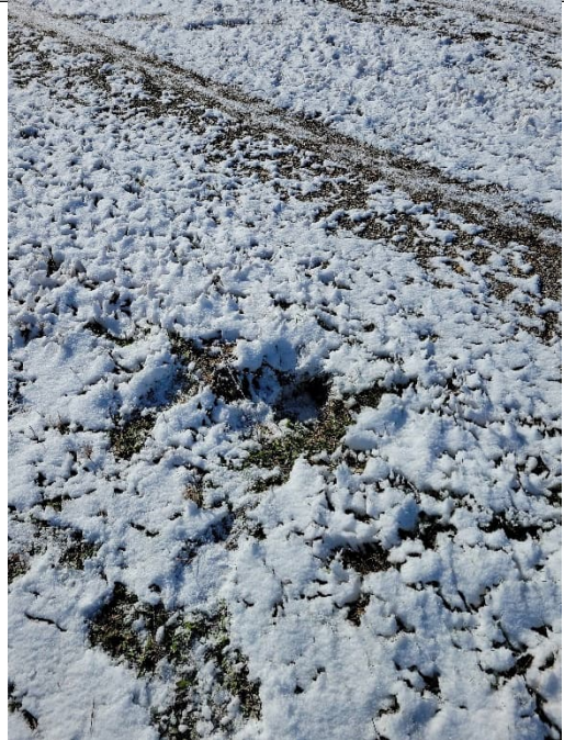
Photo 6: Animal burrow located on crest of dike near hydraulic outlet.
